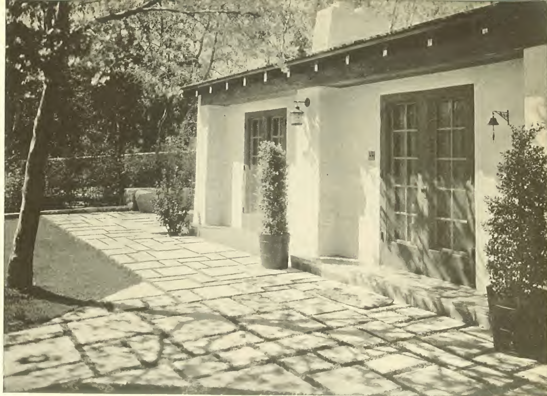
A flagstone terrace, made of concrete slabs, completes the masterpiece—a beautiful, enviable garden home. This is luxury living at low cost.
